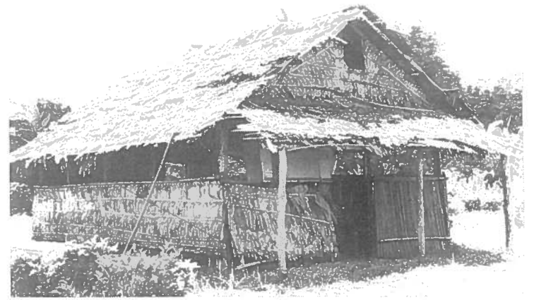
Luesalo Training Centre, exterior of our one and only classroom. Leaf buildings made of Sago palm and strips of betel nut.
