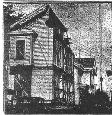
Sections underway to Meyer Park
