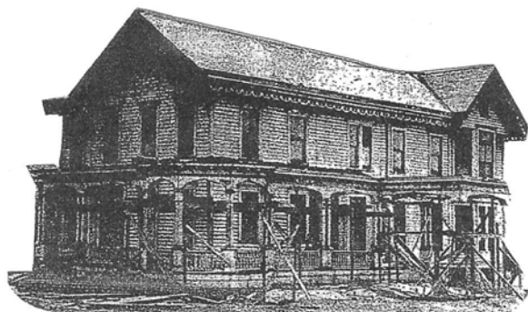
Home being reconstructed in Meyer Park
